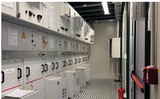
It is air-insulated, metal enclosed medium-voltage switchgear, mainly used for secondary distribution power systems. However, it is also used in special configurations for primary distribution power systems, thanks to the high rating it reaches.
