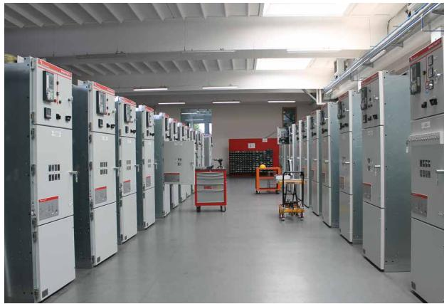
It is an AIS switchgear, fitted with metallic segregated compartments and withdrawable main components (circuit breaker, voltage transformers, protection relays). It is designed for primary distribution grids and can be supplied either in standard configuration, or as an Internal Arc-Classified IAC AFLR version. It may include the following features:
