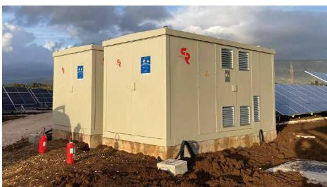
The Kiosk solution is a prefabricated plug-in compact substation, equipped with power distribution components:
