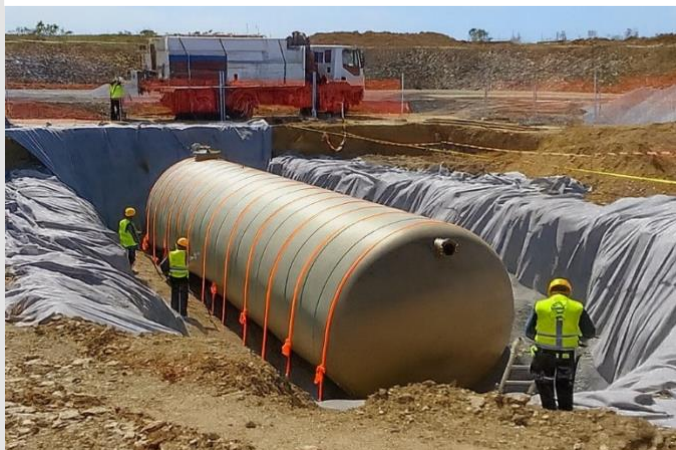
Example of installation of a DEPOSIT®-MV remote pit with 60 cubic meters of usable retention capacity.
