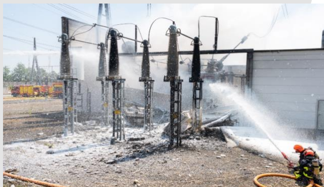
Example of foam and water spraying to extinguish a transformer fire in an electrical substation.
