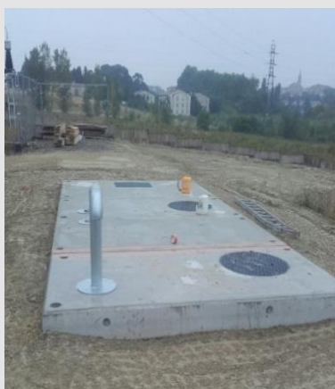
Example of prefabricated concrete remote pits or pits built on site.
