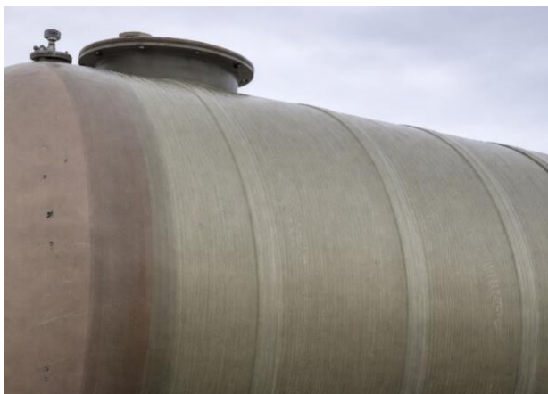
View of the positioning of the vacuum gauge and the inspection hatch.
