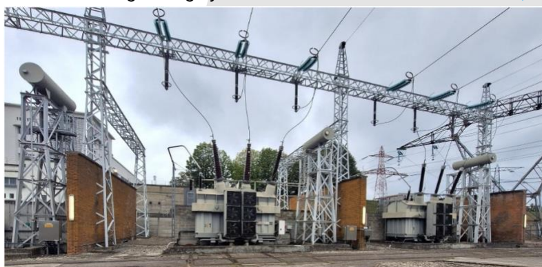
Example of several transformers with gravel-filled recovery pits directing their oils and rainwater toward a remote pit.
