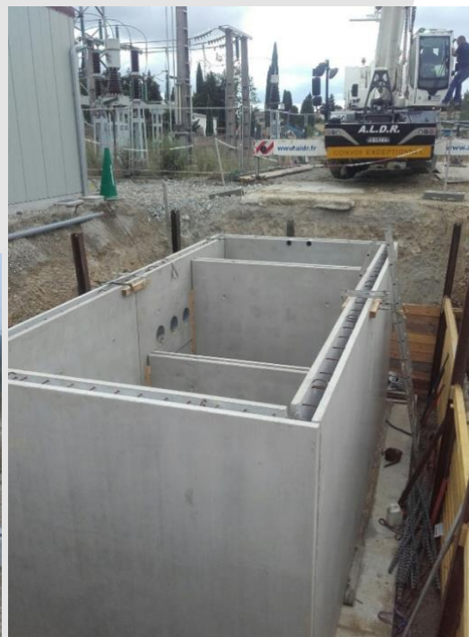
Example of prefabricated concrete remote pits or pits built on site.
