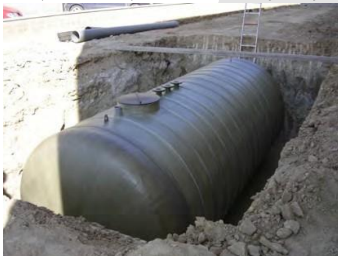
Example of DEPOSIT®-DW, or Deluge Water units, linked to fire detection systems and designed to receive large volumes of water polluted with hydrocarbons, chemicals, and similar substances.
