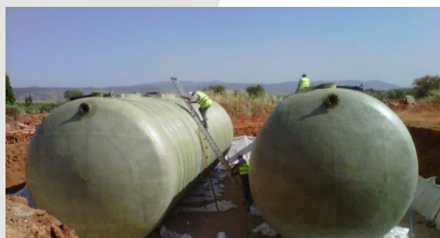
Example of two DEPOSIT®-MV 100 units, each with a retention capacity of 100 cubic meters, installed in parallel to provide a total capacity of 200 cubic meters.
