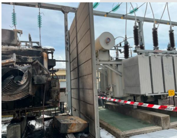
Example of passive protection : a fire wall between transformers equipped with remote pits ; only the faulty transformer was destroyed, while neighboring transformers were protected, with no oil overflow from one bay to another.
