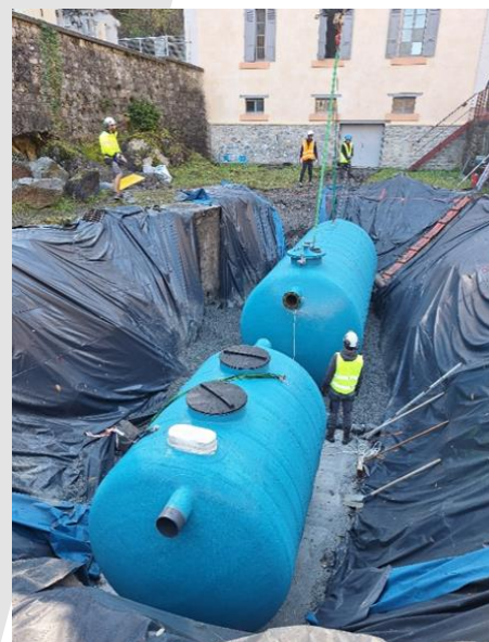
Example of a DEPOSIT®-MV with a 20 cubic meter retention capacity, equipped at the outlet with a DEPOSIT®-SEPTO hydrocarbon separator.
