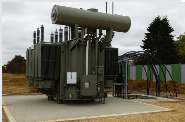
Example of a substation with a transformer installed on a concrete recovery pit, equipped with a fire-protection cover.
