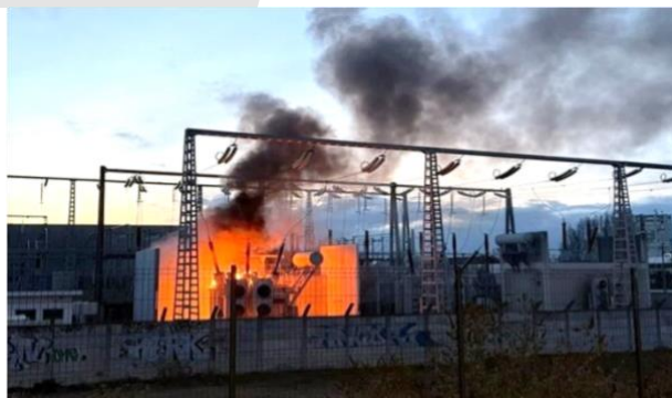
Example of an oil-filled transformer fire with hydrocarbon containment. The dielectric oil is rapidly directed toward the remote pit, reducing the risk of propagation to neighboring transformers and limiting the risk of a hydrocarbon pool fire.
