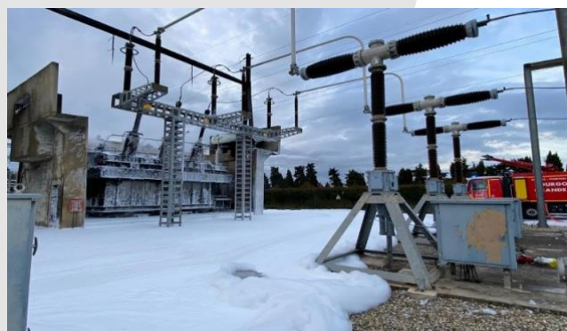
Result of foam and water spraying, illustrating the need to manage firefighting water and rainwater.
