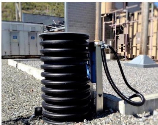
Petro Barrier Pumped PTB 24 connected to sump pump or bund guard with oil and water detection level to guarantee >5 PPM NATIONAL GRID, RTE or EON
