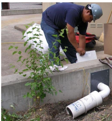
PETROPIPE PI-616-M2 alone or mounted on SANERGRID SKID 1x4 PETRO PIPE to drain by gravitation the transformer oil containment bund or concrete pit without risk of water contamination – EDF, CONEDISON or EXELON Group
