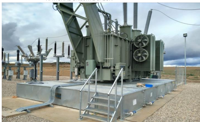
Modular Fire-Extinguishing Retention Tank ERT-MODULO 5 with access stairs and PETRO PIT-416 filtration cartridges - REPSOL
