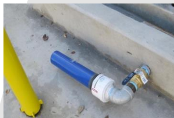
PETRO PIT 416 filter installed on a concrete retention bund
