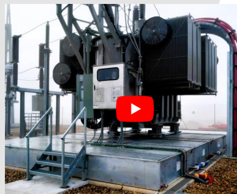
Power Transformer on SANERGRID TRT-MODULO 4 oil retention tanks equipped with SPI PIT416 drainage cartridges
