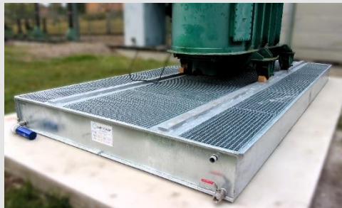
TRT®-SP equipped with raised beams, rail in order to roll the transformer and gratings for safety maintenance area
