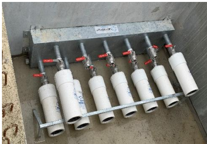
PETRO PIT 416 anti-hydrocarbon filtration kit with elbow, valve pre filter and filter connected to a ERT fire suffocating tank SANERGRID
