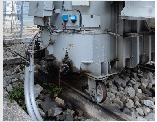
Typical oil transformer containment pit with stones and pebbles after couple of years: oil contamination, organic debris and dirt...
