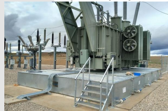
ERT-MODULO 5 tank for photovoltaic plant in remote area and need to create containment in less than 2 hours
