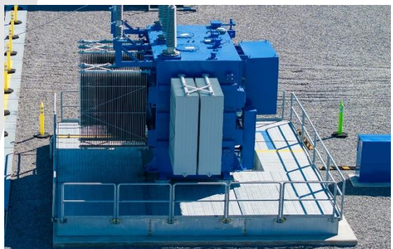
TRT-LHD-MODULO 3 retention tank with handrail equipped with filters PETRO PIPE MIDEI 7131 for synthetic oil
