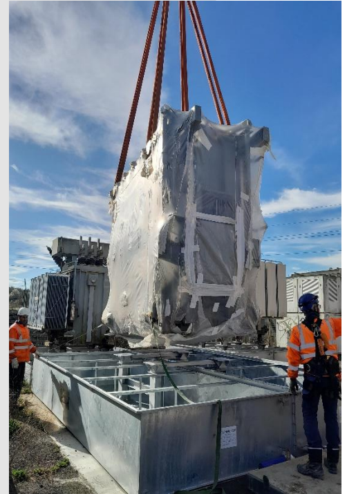
TRT®-MODUL- 2 : 2 x TRT assembled together to accept power transformer oil volume for long term storage - SNCF
