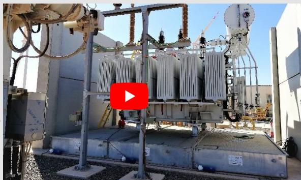
TRT®-LHD-MODULO 3 extinguishing retention tanks with rails to roll transformer on it, and SPI PETRO PIPE filtration system for mineral oil
