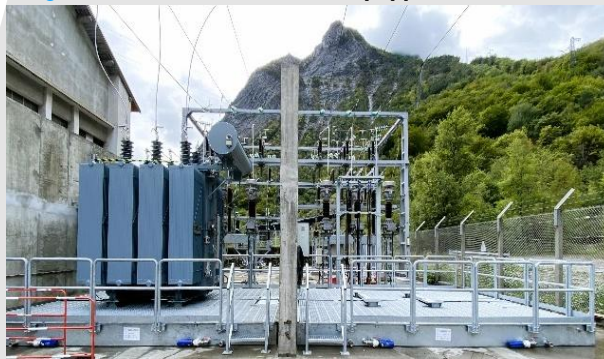
2 x ERT-MODULO 2 tank with handrail, stairs and non-slip gratings for customer that cannot dig a containment
