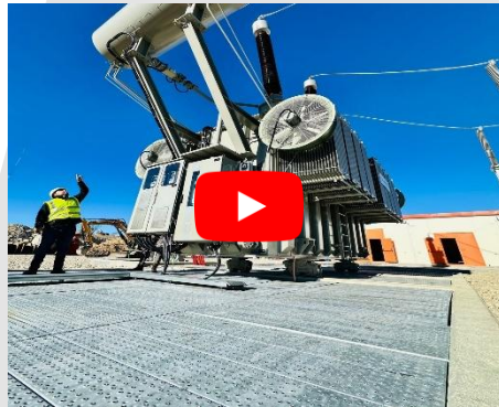
EXTICOV®-LHD® fire suffocating gratings cover, high floor resistance capacity
