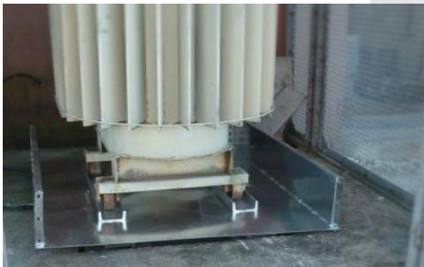
BDRG2 oil containment tank with 2 panels that can open in order to roll the transformer without use crane
