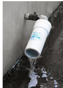
Pumped hydrocarbon filtration system PETRO-BARRIER
